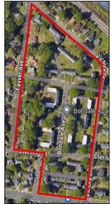
Figure 16. Aerial View of Bondale Apartments (Image Source: Google Maps)
