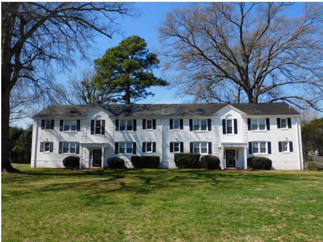
Figure 17. Representative Apartment Buildings at Bondale Apartments (Image Source: Commonwealth Preservation Group, 2024)
