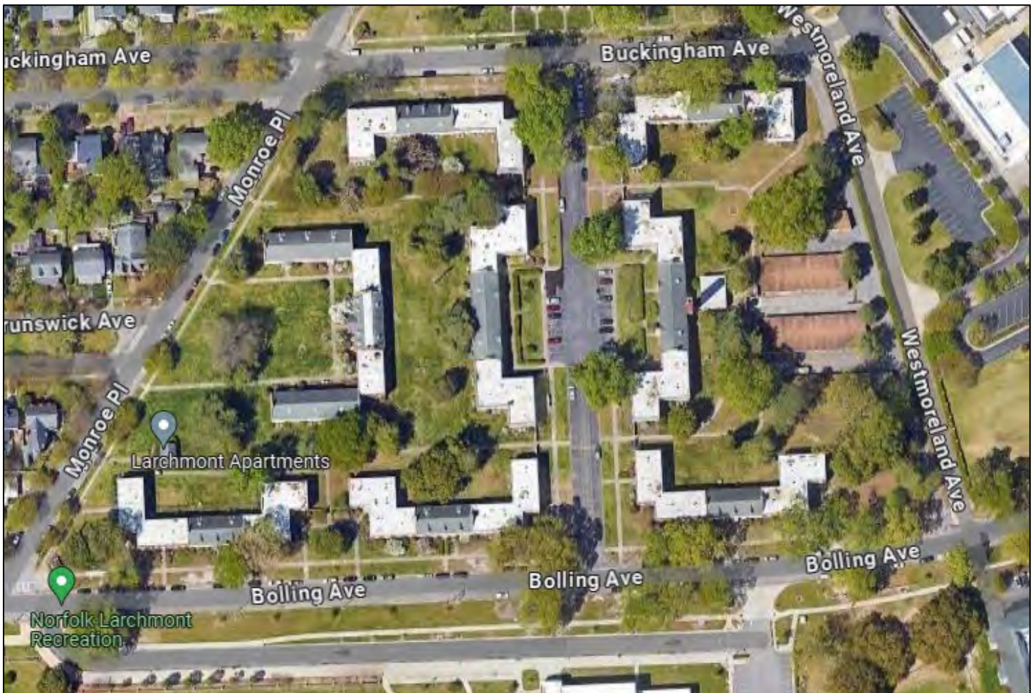
Figure 3. 2024 Aerial View of Larchmont Village Apartments (Image Source: Google Maps). The site plan and landscape design display character-defining features of garden apartment complexes, including ample space between buildings to provide residents with easy access to the outdoors, a parking lot concealed within the complex's interior, ample vegetation, and emphasis on walkability via a paved circulation network within the complex that also linked it to the surrounding neighborhood.
