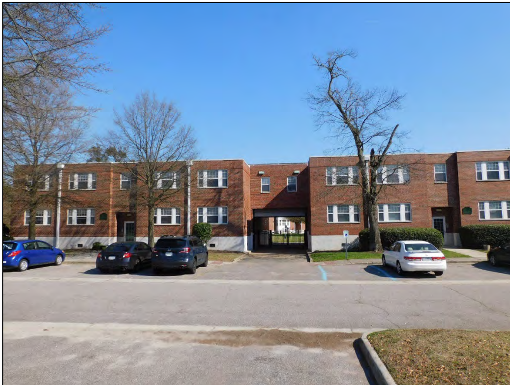
Figure 28. Representative Apartment Buildings at Kingsley Lane Apartments (Image Source: Commonwealth Preservation Group, 2024)
