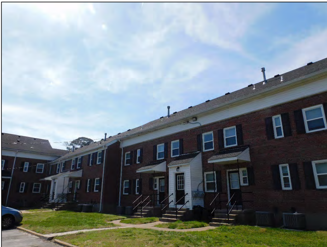
Figure 23. Representative Apartment Buildings at Sussex-at-Norfolk (Image Source: Commonwealth Preservation Group, 2024)
