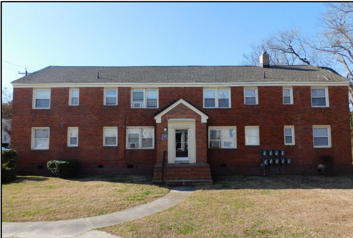
Figure 6: Building Type F Example – 302 Warren Street (CPG)
