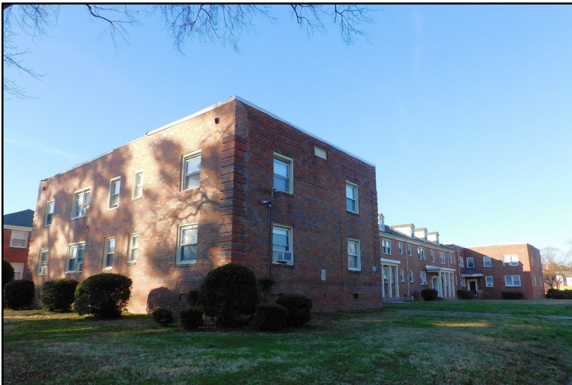
Figure 12: Building Type L Example – 7205 Remsen Street (CPG)
