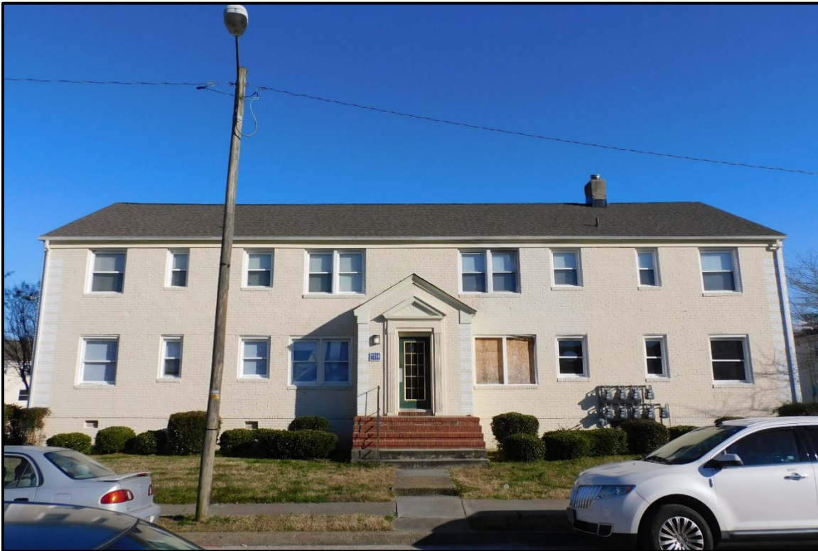
Figure 11: Building Type K Example – 7218 Ralph Street (CPG)
