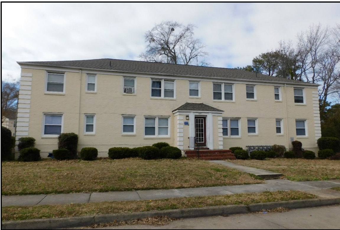
Figure 3: Building Type C Example – 7277 Remsen Street (CPG)
