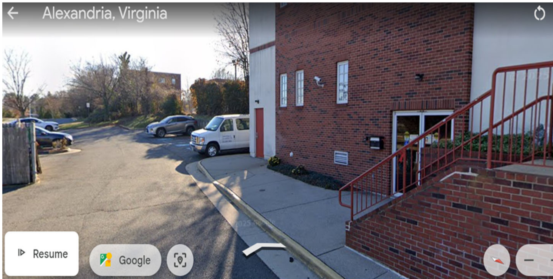
Photograph 7 - East Side of Church
