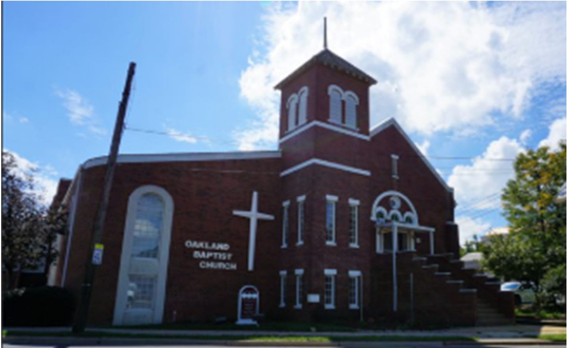
Photograph 1 - Picture of Renovated church 1999.
