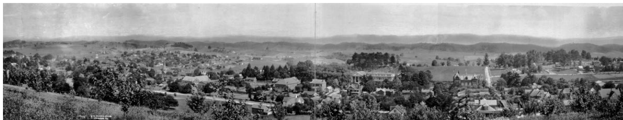
Figure 13. Birdseye view of Abingdon in 1915.
