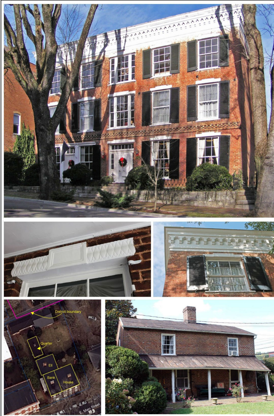
Figure 4. Abingdon Bank (140-0037-0053; 225 East Main Street), clockwise from top: facade in 2005; cornice and window detail in 2023; quarter in 2023; layout of bank/house, ell, quarter, and yard; window lintel detail in 2023 (all photographs by Michael Pulice, VDHR).
